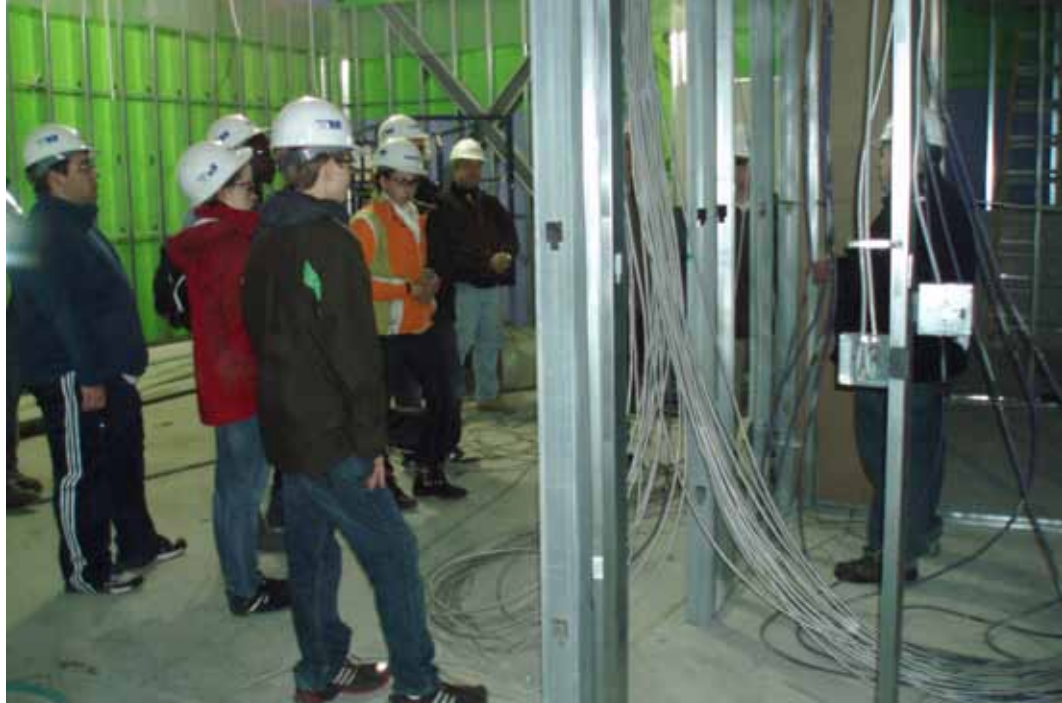
Portland High School students tour a local restaurant during construction. Photo courtesy of Jill Simpson, AIA.
